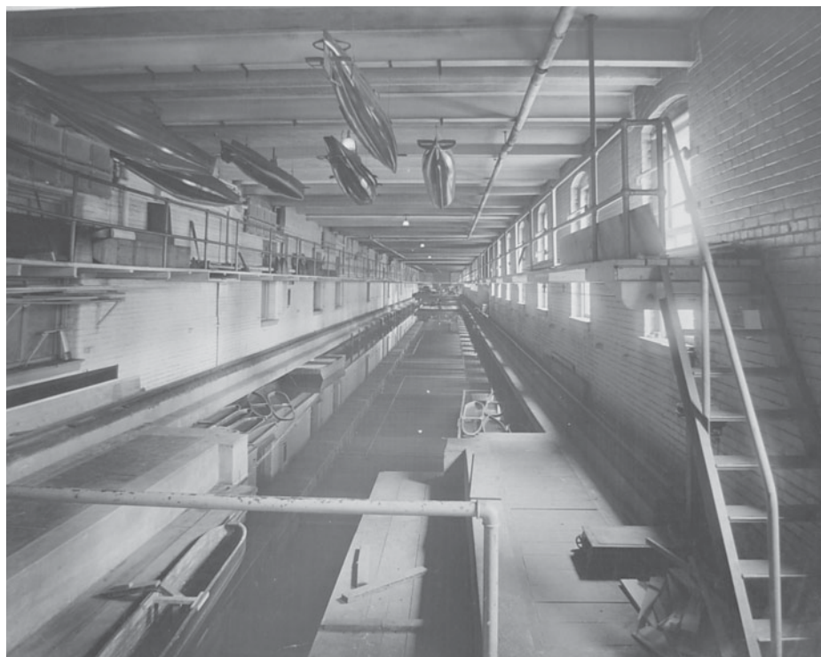
Figure 3. The test tank in the new engineering building at the University of Michigan. Cooley Papers, Bentley Historical Library, University of Michigan, Box 66.
