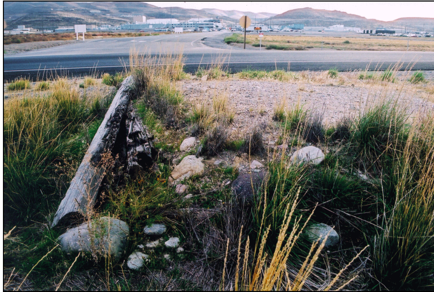
Figure 5. North wall of bunk house at Kolmar Station (Lampo). Taken from Lampo Site Form (42BO1148). (Photograph courtesy Commonwealth Heritage Group.)
