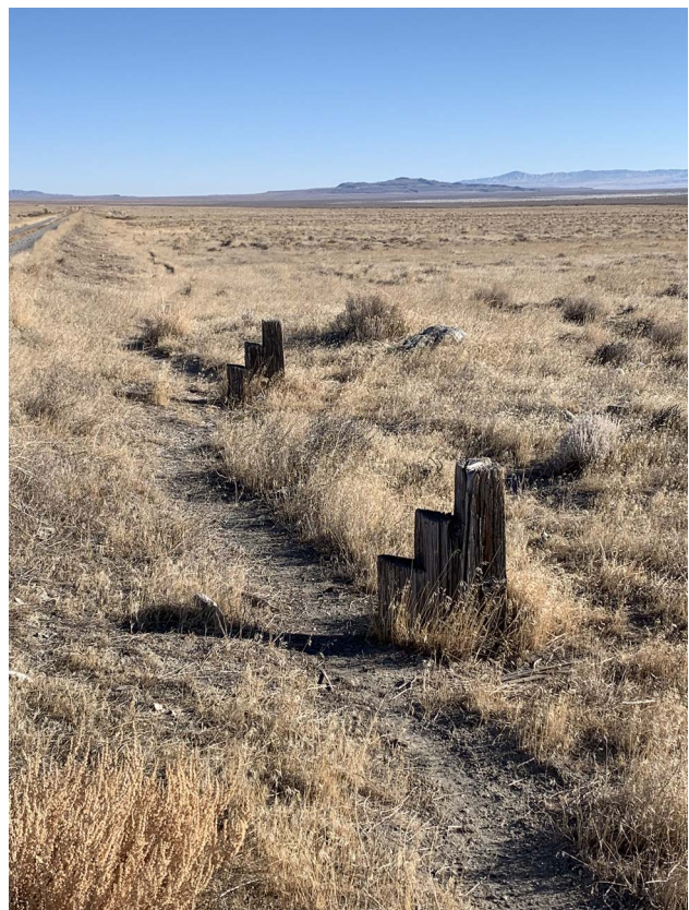
Figure 1. A rail rest feature located on Central Pacific (CP) line east of Lucin in Box Elder County, Utah. View to the east toward Terrace. Note railroad berm on extreme left of photograph. (Photograph by Chris Merritt, December 2020.)
