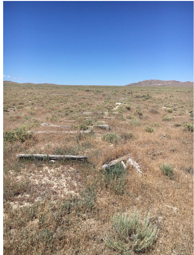
Figure 2. Railroad berm on the abandoned railroad wye at Matlin, Utah. The desert environment has preserved many crossties on the berm 79 years after abandonment. (Photograph by the author, 2019.)
