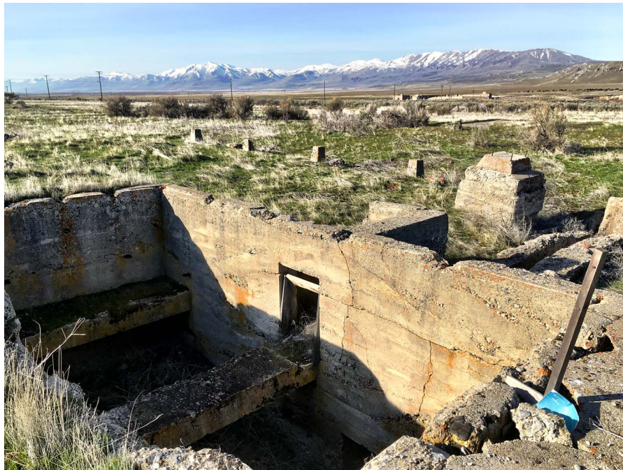
Figure 6. Warehouse foundation at Lampo Station. (Photograph by Chris Merritt.)
