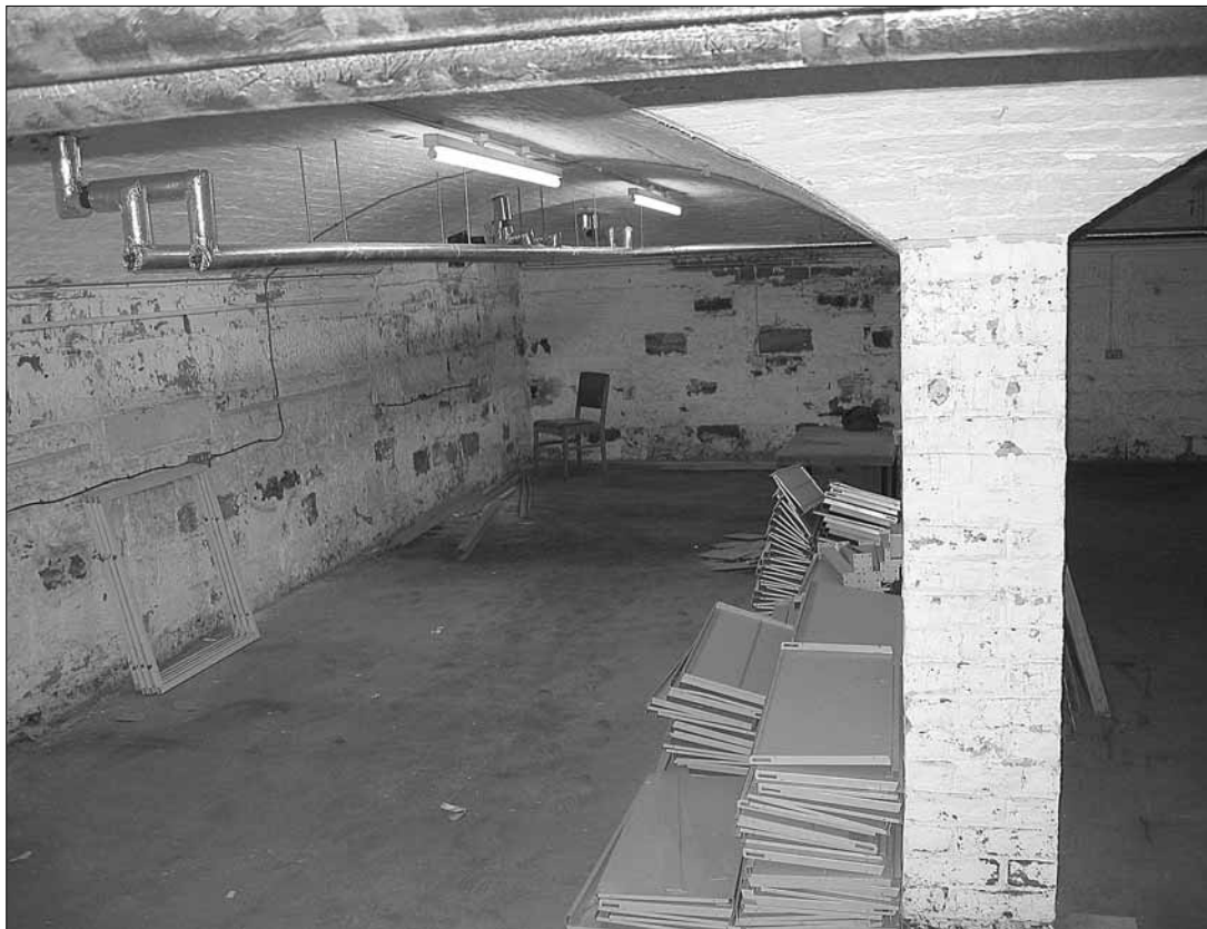
The basement site: the vaulted wine-cellar. Photo: V. Hunter.
