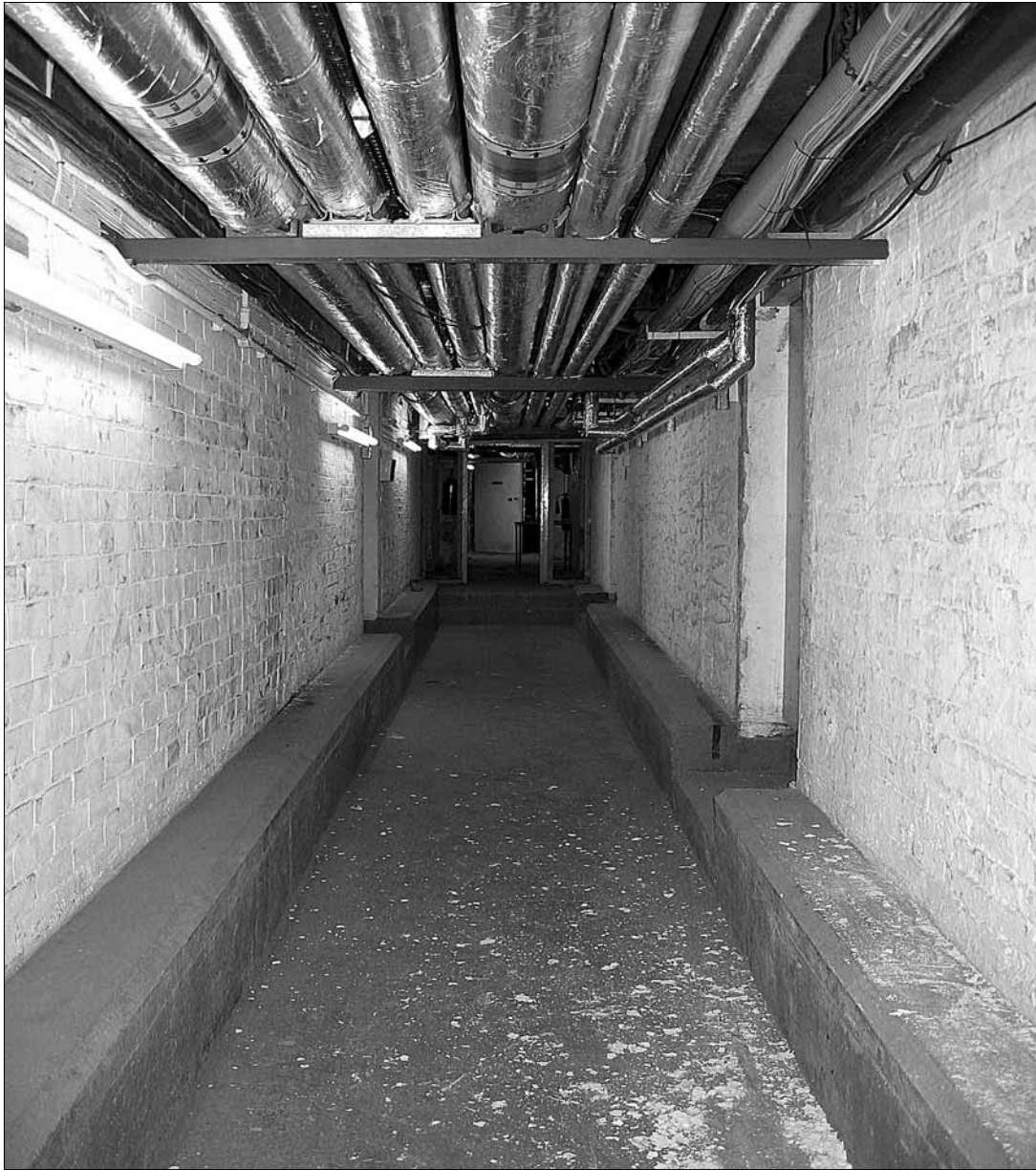
The basement site: the service corridor. Photo: V. Hunter.
