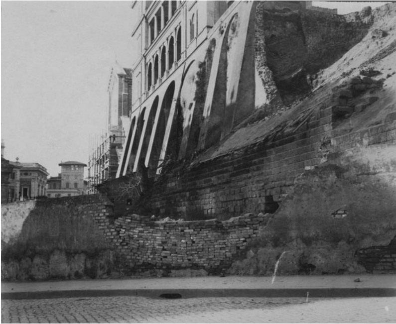
Fig. 12. Photograph by E.B. Van Deman taken during the destruction of the Villa Spithöver showing the original extent of the ashlar wall beneath. American Academy in Rome, Photographic Archive, Van Deman Collection no. 86/188. (Reproduced courtesy of the American Academy in Rome.)
