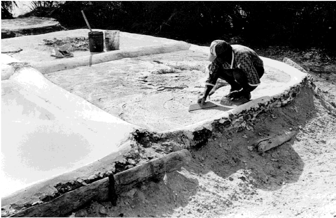
Figure 5. The sand mixed with lime is being applied to the surface of the era using a wooden slat, or paleta .
