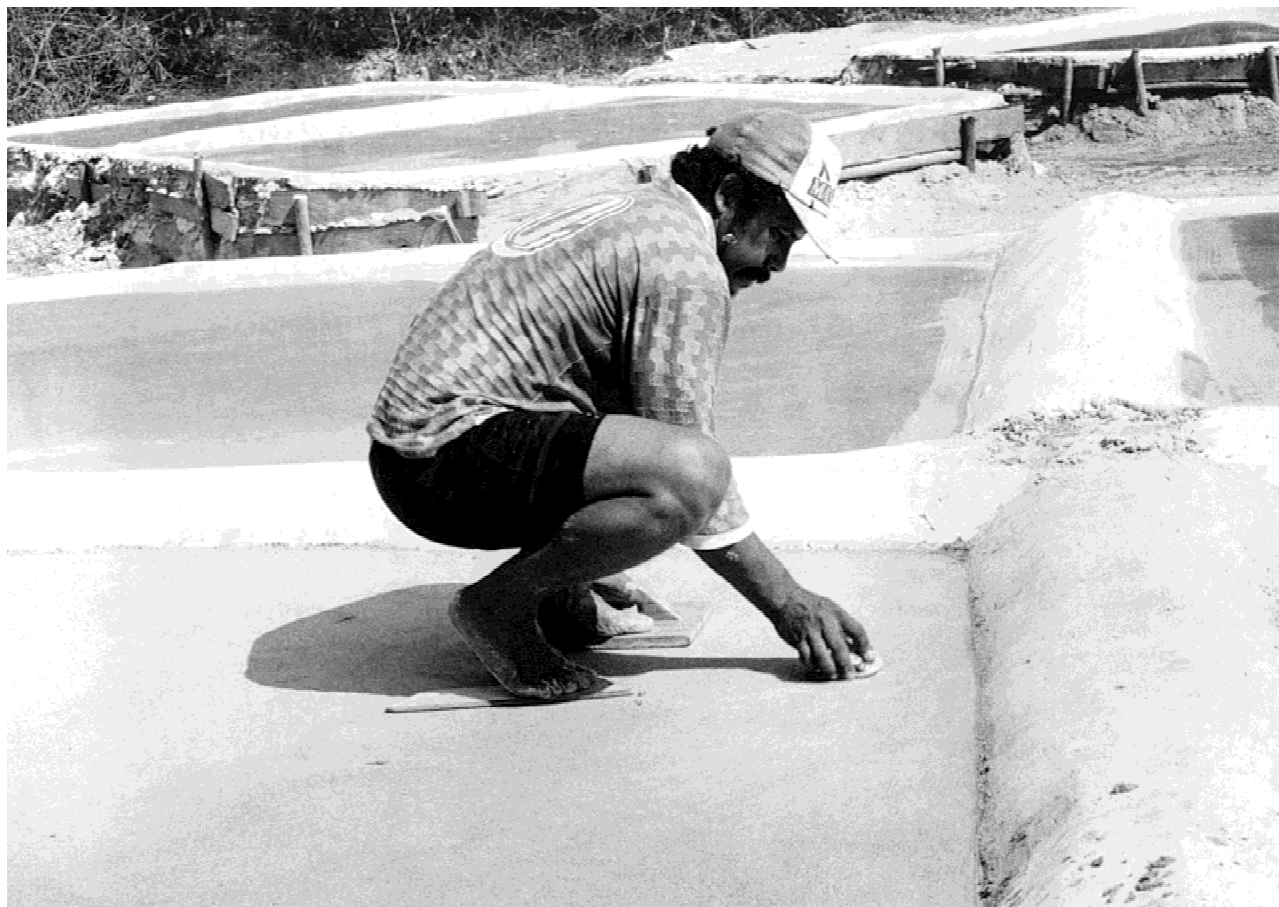
Figure 7. The surface of the era is polished with a stone to make it smooth and more compact, thus averting leaks.
