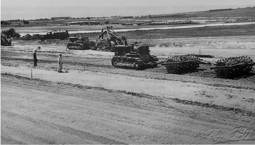
Figure 2. Soil compaction of the reinforced concrete runway at Yeşilköy Airport, c.1950. Sarıgöl, op. cit., p. 104 (used with permission).
