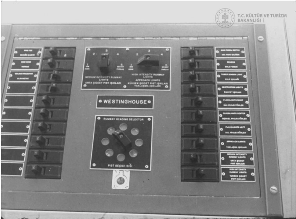
Figure 6. A close-up view of the Westinghouse equipment in the air traffic control tower at Yeşilköy Airport, 1953. The Ministry of Culture and Tourism of the Republic of Türkiye (used with permission).
