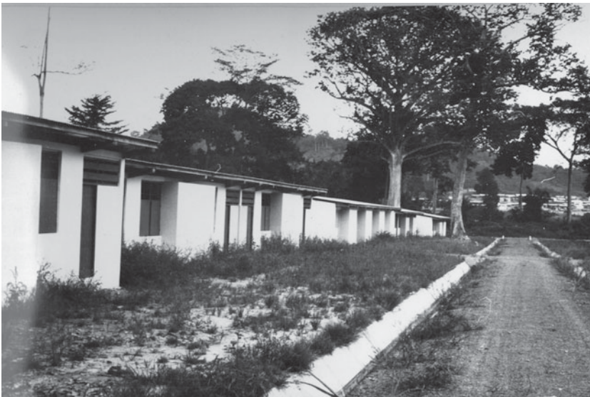
Fig. 3. Workers' housing, Akosombo Community 2; Ghana vol. 46, DIARY-GHA 3, Dec. 1963, 16 (Archive files 24477), Constantinos A. Doxiadis Archives, © Constantinos and Emma Doxiadis Foundation.
