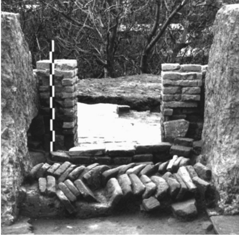
Fig. 4. Collapsed arches of the main entrance viewed from the inside of the church. Reproduced after Savchenko, 2005.
