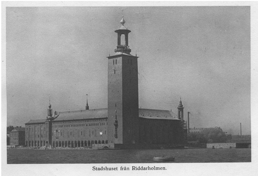
Figure 2: The city hall of Stockholm (1923) derives its monumentality from its detachment from the old city centre. Like all modern city halls, Östberg's city hall is also a dual-purpose building with a representative side and an administrative side. The building follows a rectangular ground plan, built around two open spaces. It is a piece of art, planned to be viewed from a distance. The water, the tower and the spacious layout create the illusion of monumental, but romantic sacredness. Source: Stockholms stadshus, 1923.
