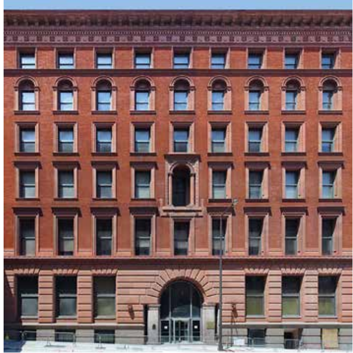
Fig. 14. Endicott Building, St Paul, Minnesota, Gilbert & Taylor, 1889–90, Fourth Street facade, photograph by David Enblom, 2012
