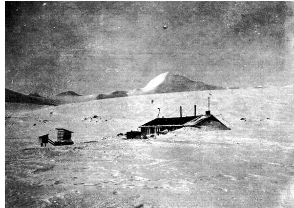
Fig. 5. 'Casa Moneta', Laurie Island, South Orkney Islands. Built in 1905, the oldest continuously used building in the Antarctic photographed about 1920. (photograph provided by Tutta Holtan)
