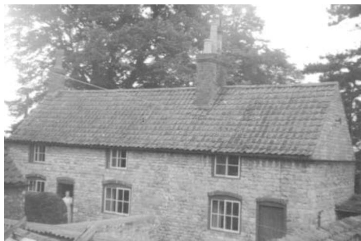
Figure 8. The head gardener's house (HG on Figure 4), built as two cottages by the churchwardens in 1797 for £118 1s 7d. Stone and pantile, typical of the pre-1860 period (photo, 1956, Dennis Mills).
