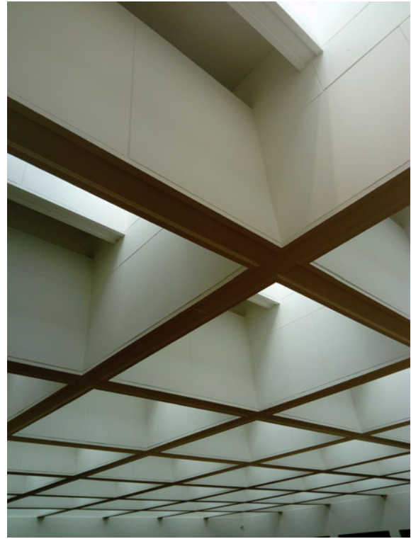
Figure 12: Internal view of the restored panels.
