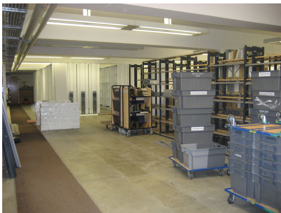
Figure 2: Dismantling of the old shelves and preparing for the new.
