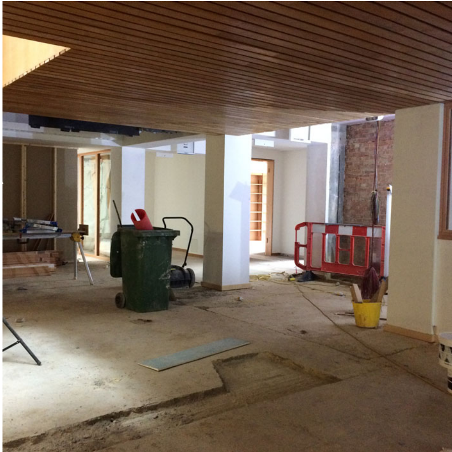
Figure 4: Demolition of the old enquiry desk area.
