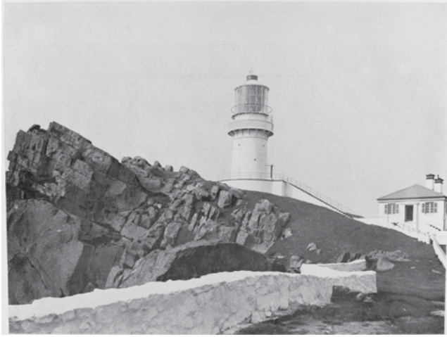
Fig. 3. Peiyüshan Lighthouse in situ, c. 1932.
