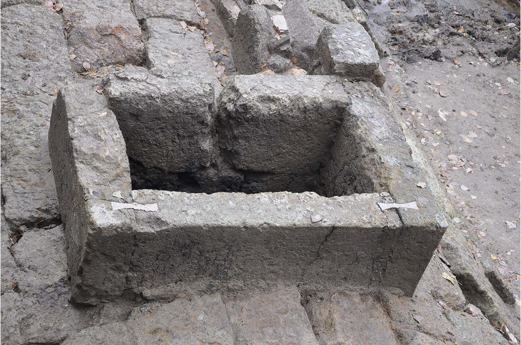
Figure 9. One of the two access openings, with the dovetail clamps surrounded by lead, and a rope-wear groove on the far side of the opening (photograph by P. Popović & A. Djordjević).
