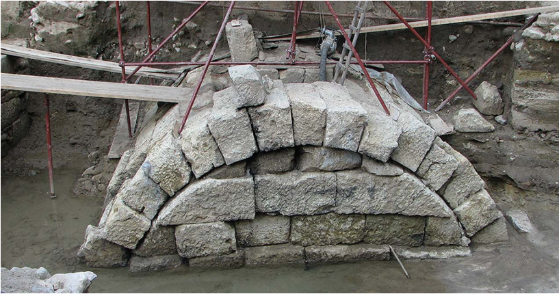
Figure 2. Left) photograph of the Kale-Krševica barrel-vaulted reservoir (and supporting scaffolding) taken during excavation and showing the extent of waterlogging; right) profile drawing (photograph by P. Popović & A. Djordjević; illustration by N. Lazarević).
