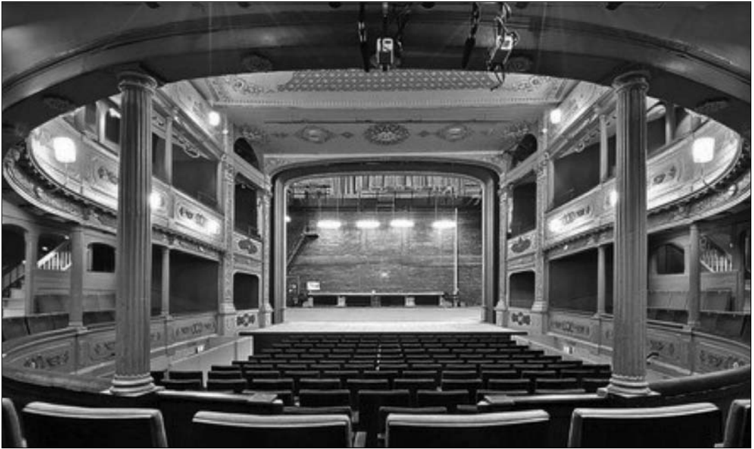
Paty's Doric columns: 'as slender and as widely spaced as possible to maximize sightlines'.
