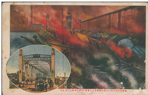
Figure 10. Taishō 12. 9. 1 (Great Tokyo Earthquake) Pitiful Azumabashi Bridge Destroyed by Fire and Before the Quake.
