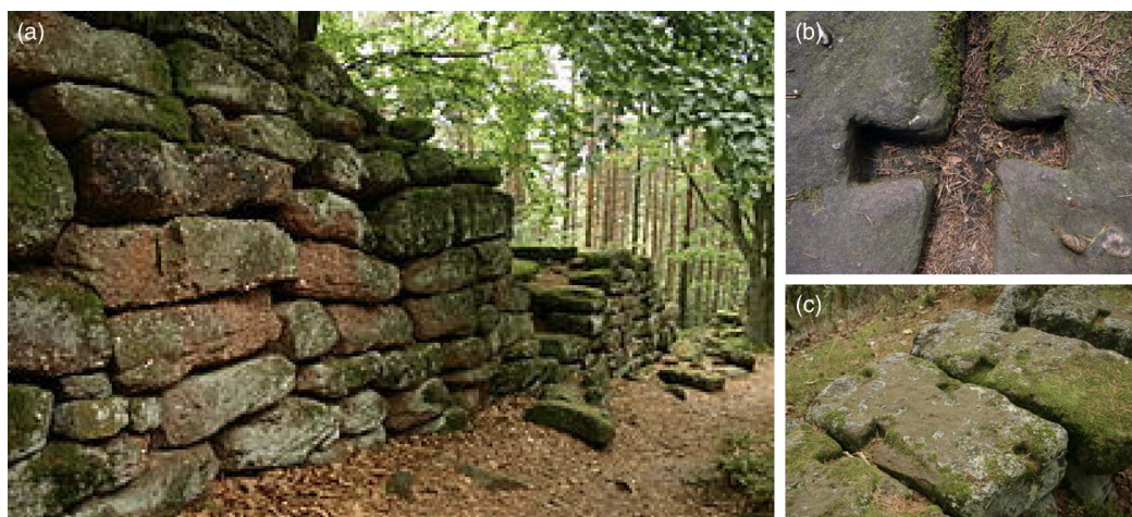
Figure 4 Strasbourg, Mont Sainte Odile (France), Mur Païen: (a) a well-preserved stretch of the “Pagan Wall”; the individual ashlars are approximately 50 cm in height; (b) exposed layer of worked stone blocks on outer face of the wall shows recipients for tenon joints; (c) detail of corresponding cut out cavities with characteristic dove-tailed shape.
