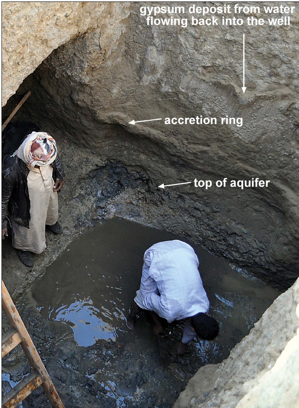
Figure 7. Accretion ring and top of the aquifer on the well's western wall (photograph by M. Woźniak).
