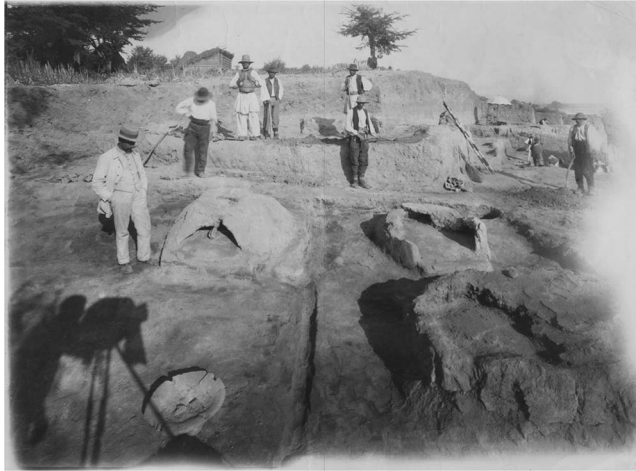
Figure 15 Miloje Vasić (left) supervising the excavation and recording of a house at 2.91 m in 1911.
