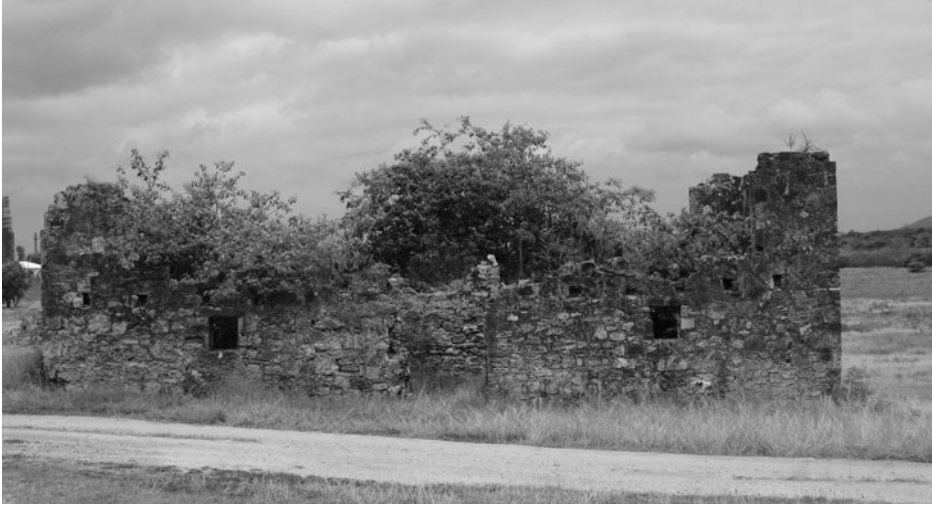
Figure 2. Cane Garden hospital building, facing west (photo by author).
