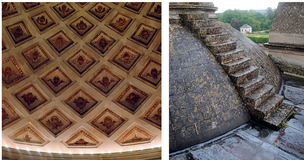
Fig. 14. Details of the dome's surfaces of intrados (left) and extrados (right) showing the joint lines and the progressively diminishing size of its stone courses (photographs by the author)
