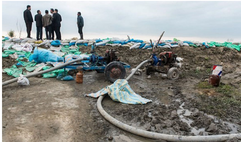
The Embankment Made of Bags of Mud and Sand Around Haji-Abad.
