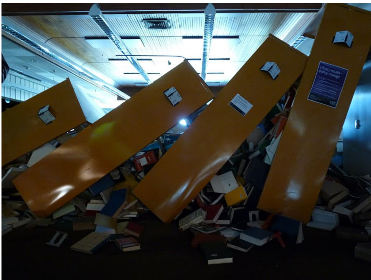
Figure 1: Collapsed shelves in the Central Library. Photo: University of Canterbury
