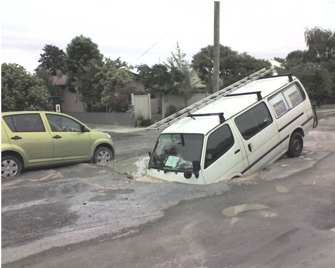
Figure 4: Sink holes in a road caused by liquefaction. Photo: Matthew Journee, used with permission
