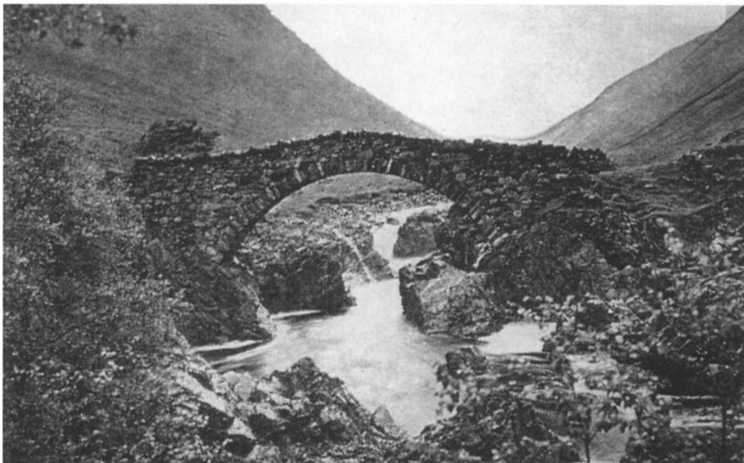
Figure 2 Dail-an-eas [Waterfall] Bridge, Glen Tilt – the bridge is now in ruins.
