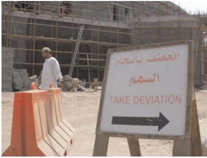
Figure 1. 'Detour' sign at construction site – Sohar, Oman
