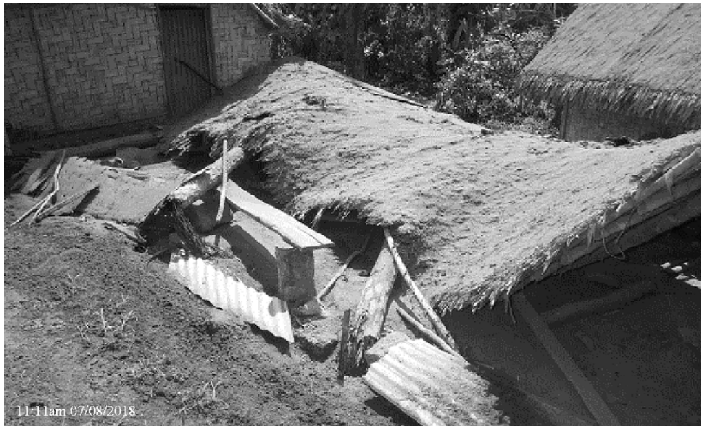
Figure 4. Village Well Contaminated with Ashfall after Protective Metal Sheets Collapsed, South Ambae.
