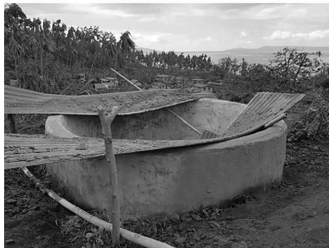
Figure 3. Complete Collapse of an Open-Sided Traditional Building (55mm ashfall depth).
