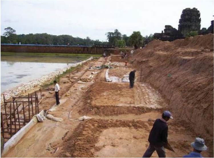
Figure 6. The moat repair in 2003/2004 displays the massive buried clay embankment (image courtesy of Valter Santoro 2005).
