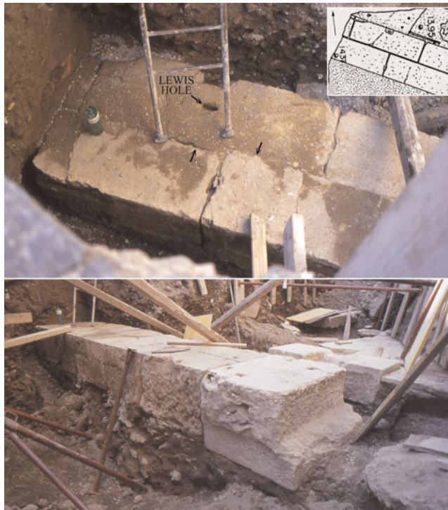
Fig. 8. The squared-stone masonry, showing the misaligned joints (note the arrows) and the only hole for lewis irons (above), not recorded by Vitti (inset: cf. Fig. 2), and the foundation of the ashlar wall (below). (Photos: author.)
