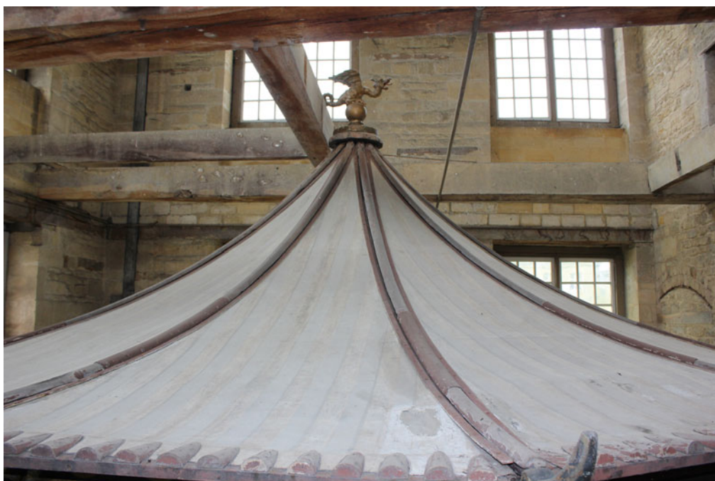
Fig. 7. The Chinese Pavilion, Boughton, Northamptonshire, view of the striped roof covering
