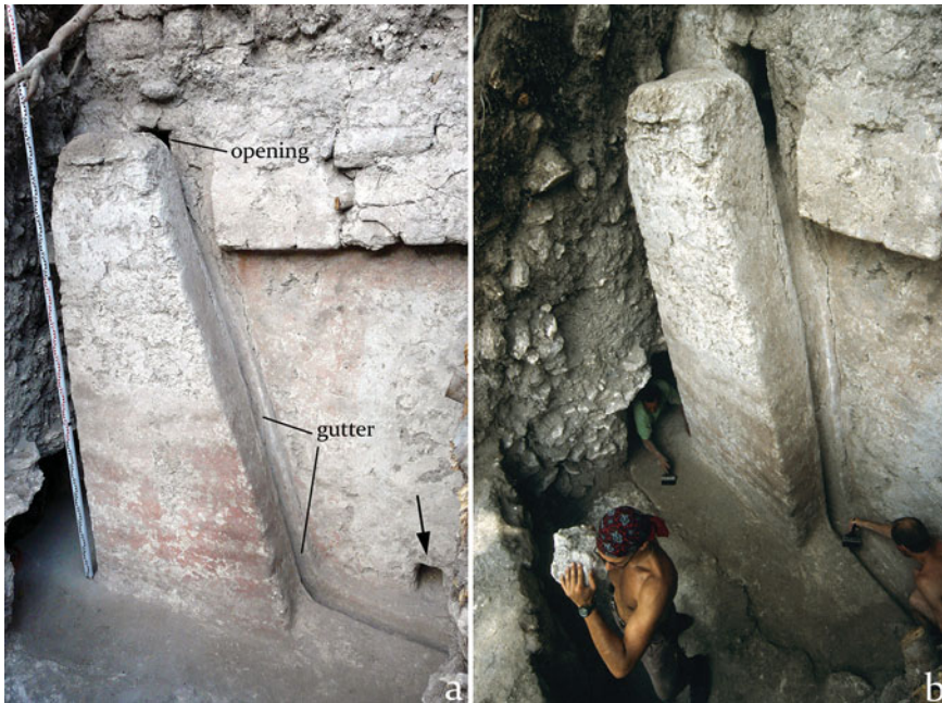
Figure 9. Trapezoidal element attached to the wall with the drain—a possible replica of a sacred mountain (note the opening on the exterior of the wall through which water comes). Located in the lower part of the wall and marked with an arrow is the aperture that served to drain the passageway located behind the wall (photographs: Wiesław Koszkuł and Robert Słaboński).
