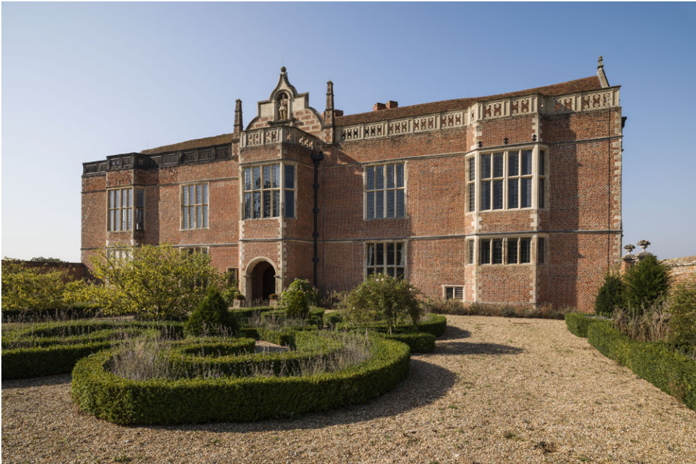
Fig 21. Bramshill's east front, with gatehouse on the ground floor, long gallery on the first floor and access to the southerly roof walk above. Photograph: © Historic England Archive, DP184529, reproduced with permission.
