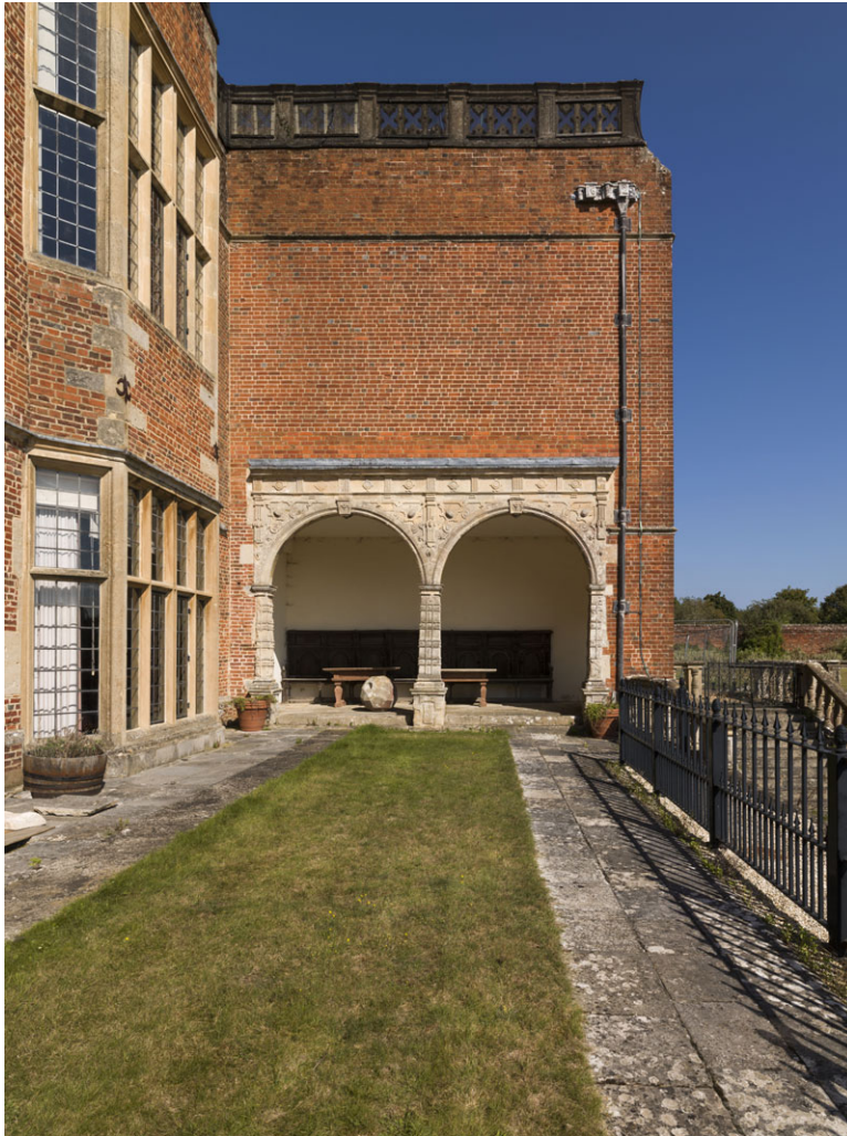
Fig 29. The loggia on the east side of Bramshill's south terrace, believed to have been installed in this location around the early eighteenth century. Photograph: © Historic England Archive, DP184548, reproduced with permission.
