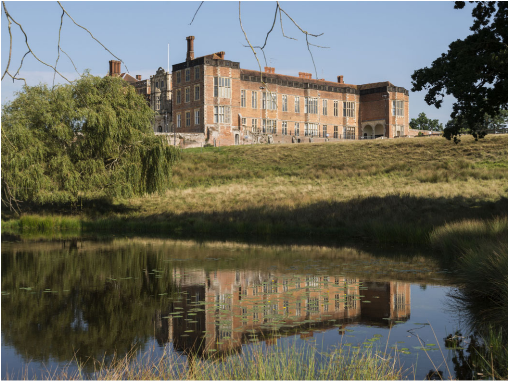
Fig 1. Bramshill viewed from the south-west in 2016. Photograph: © Historic England Archive, DP184539, reproduced with permission.
