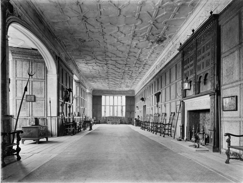
Fig 17. Bramshill's long gallery, nearly 130ft (40m) in length, in a photograph of 1923. The ceiling is Jacobean, but the panelling is believed to date from later in the seventeenth century.
