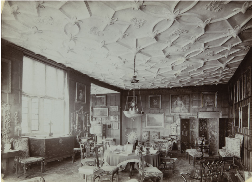
Fig 23. The great chamber over the hall (Chapel Drawing Room), in a photograph of c 1910. The plaster ceiling dates from c 1607. Image : Historic England Archive, ref. OP28108, reproduced with permission.
