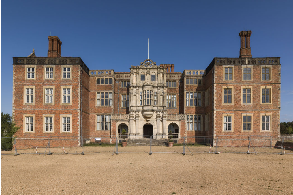
Fig 4. The west elevation of Bramshill in 2016. The stone frontispiece was built in 1612 or shortly afterwards. Wings that originally projected to each side were demolished in about 1703. Photograph: © Historic England Archive, DPI84533, reproduced with permission.
