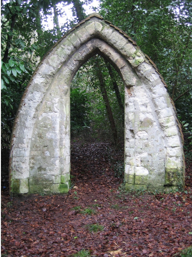
Fig 11. Internal window rere-arch from the 7 Ireland Yard building, re-erected in 1900 in the grounds of Selsdon Park, Croydon. Photograph: the authors.
