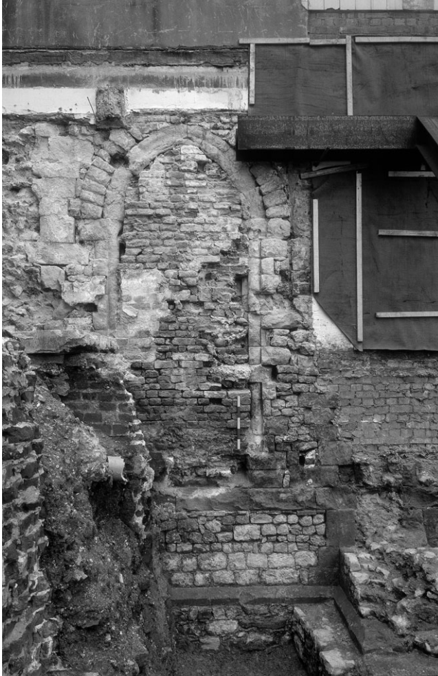
Fig 12. View of the external window arch, discovered in the 10 Friar Street excavation in 1988.
