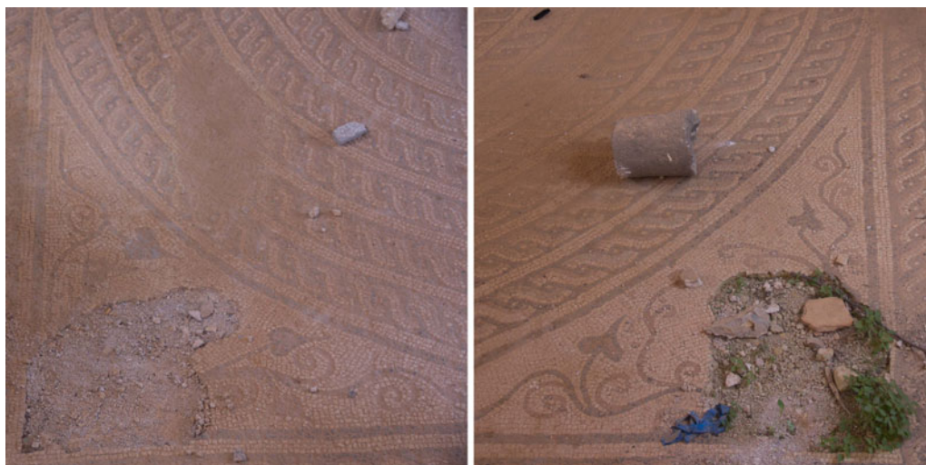
Figure 4. Details of the removed spandrels, Spring to the left and Winter to the right, the Seasons mosaic, House of Jason Magnus, Cyrene. Photograph: W.T. Wootton.
