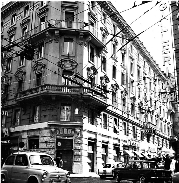
Fig. 2. Rome, 45 Via De Pretis, the headquarters of SGI from 1926 to 1966, photograph of 1964 (Central State Archive, Rome)
