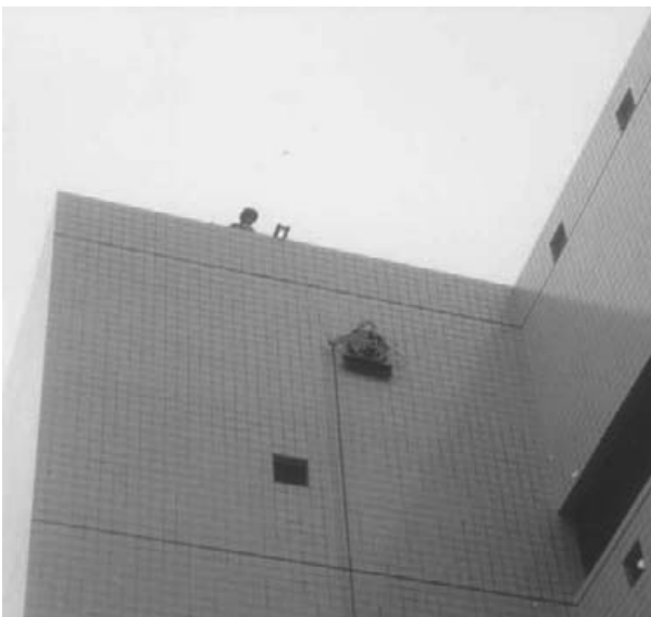
Fig. 8. Photo of robot cleaning the ceramic tile surface.
