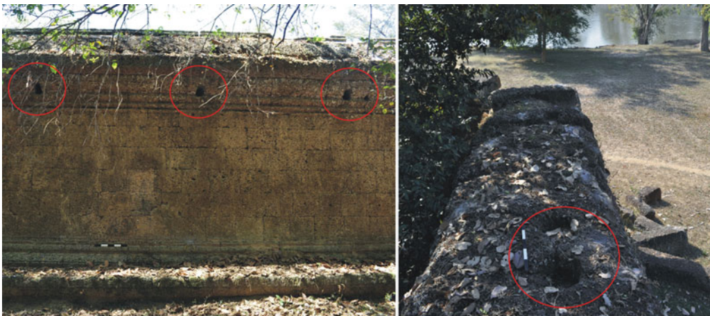
Figure 2. The fourth enclosure wall of Angkor Wat showing the horizontal holes on the inside face (left) and vertical holes along the top (right).
