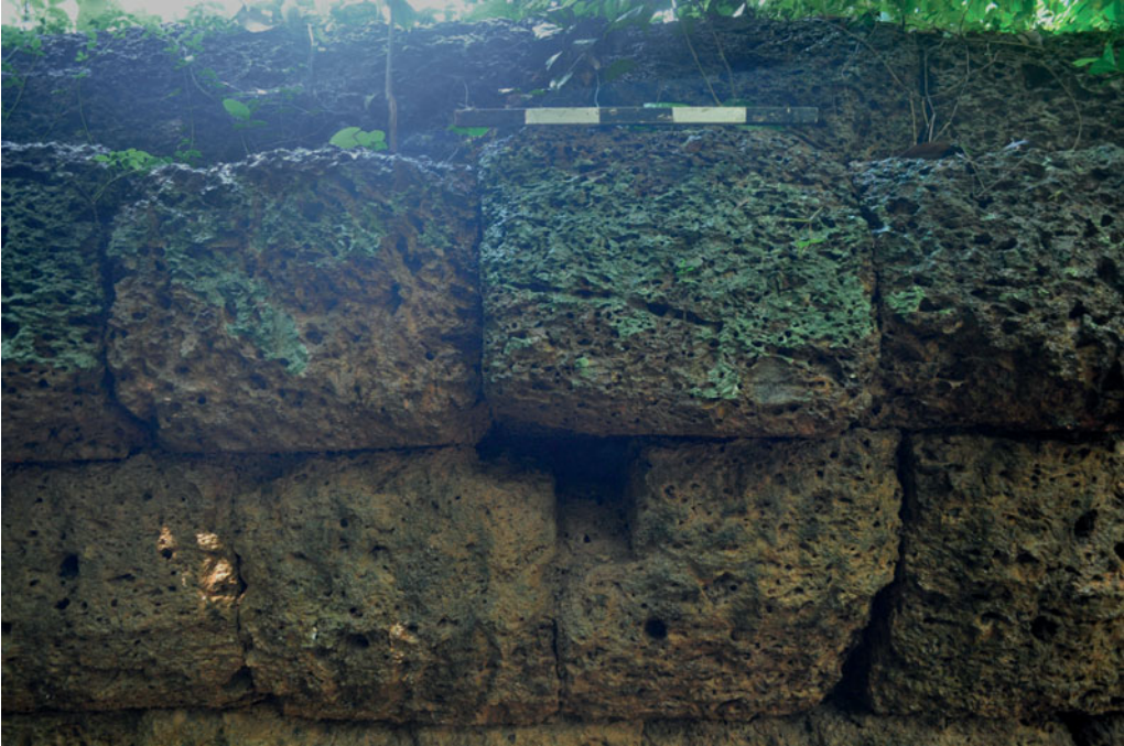
Figure 11. Irregular hole located to the upper left of a regular hole, forming an inverted L-shape.
