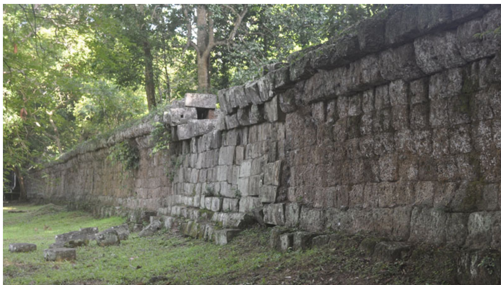
Figure 4. Gateway gap on the south wall, east side, exterior.
