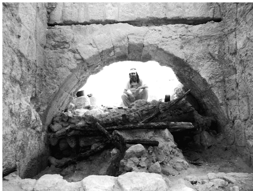
Fig. 22. Wooden reinforcement of the retaining wall of the Bar-Kokhba Revolt (view from north) below the passageway's S vault (© Herodium Expedition, R. Porat).
