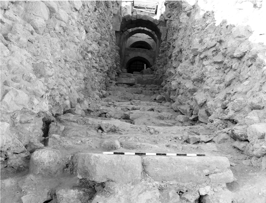
Fig. 13. View of the stepped foundation in the area to the north of the arched passageway, with the in situ stone step in the foreground (© S. Tiram).
