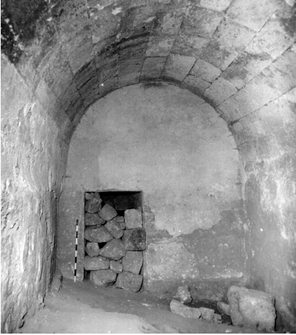
Fig. 5. Vaulted room below entrance room, with doorway to curvilinear corridor (view from east) (© G. Foerster).
