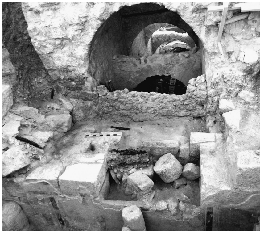
Fig. 21. Retaining wall (partly dismantled) datable to the Bar-Kokhba Revolt, built below the S vault of the passageway (view from south) (© Herodium Expedition, R. Porat).
