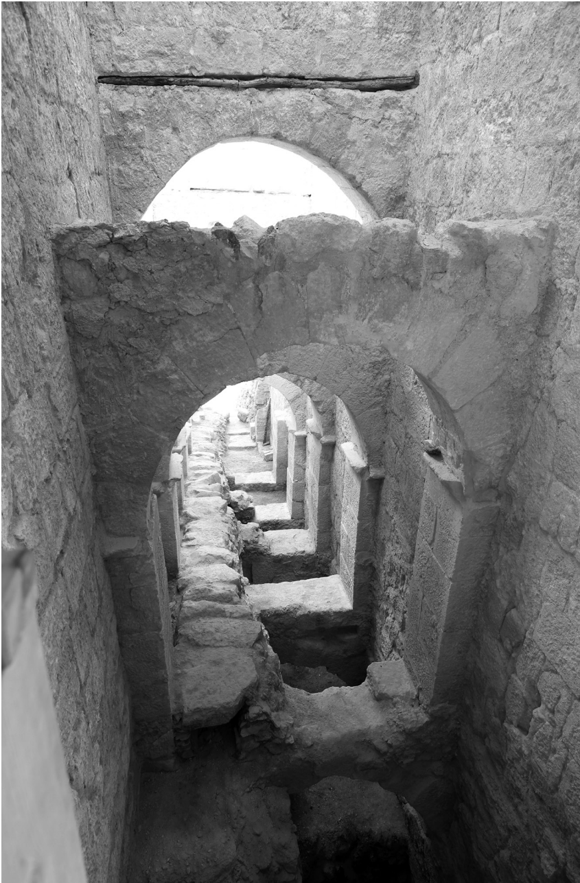
Fig. 15. The drainage channel built along the passageway's W wall (view from south) (© S. Tiram).
