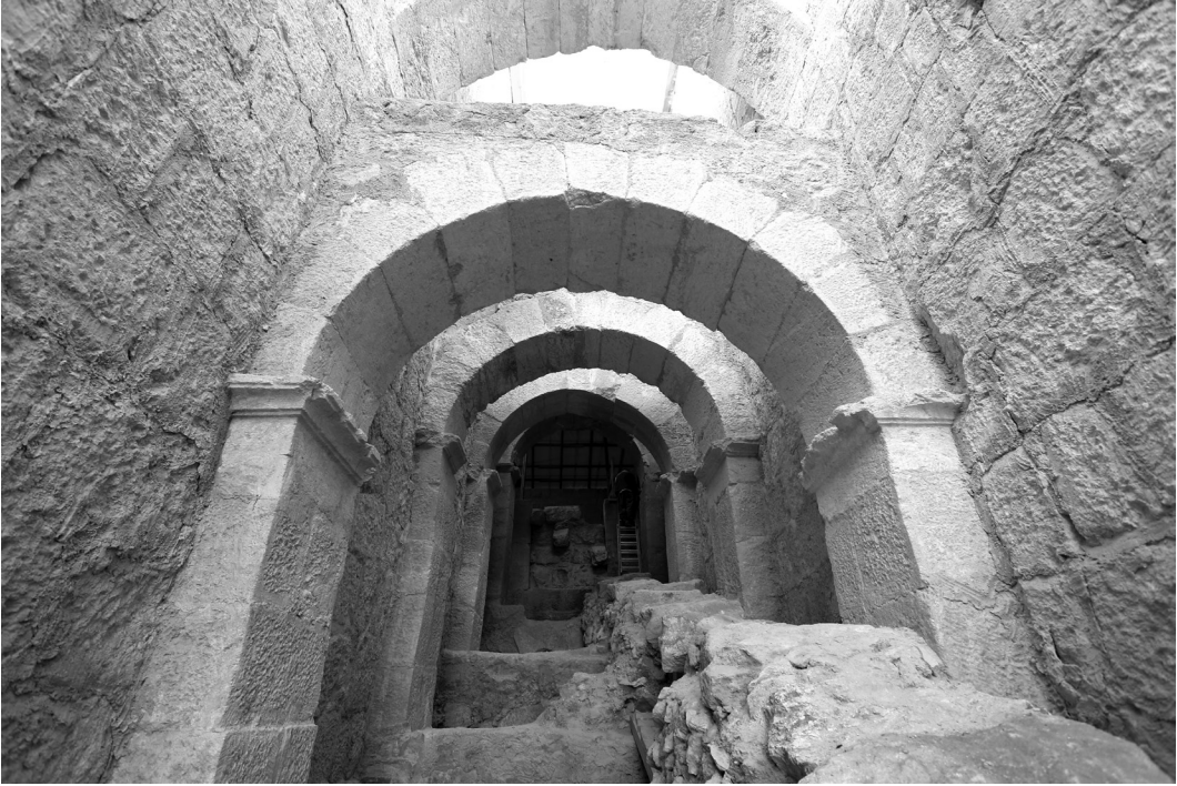
Fig. 10. The arched passageway as seen from within (view from northeast) (© S. Tiram).
