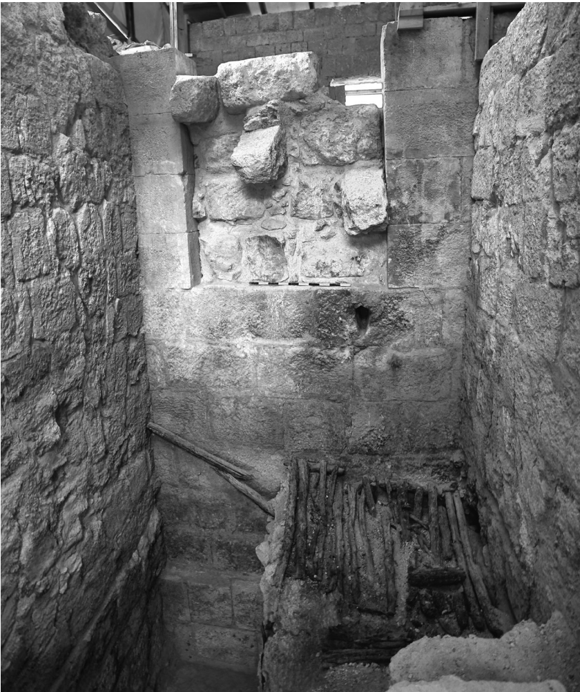
Fig. 24. Roof of tunnel of the Bar Kokhba Revolt, with numerous wooden beams laid horizontally side by side, as preserved in situ . Note the blocked entrance doorway to the mountain palace (top) (© S. Tiram).
