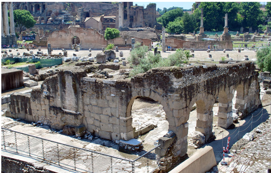
Fig. 14. View from the northeast of the 9th-c. domus solarate within the Forum of Nerva. Note the arcuated portico lining the early medieval cobbled street on the northern (right) side of the structure. (M. Andrews.)
