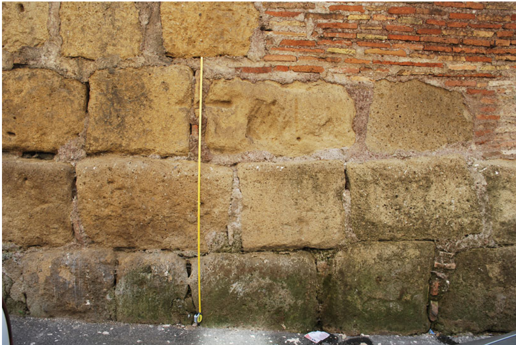
Fig. 1. Reused ancient tuff blocks on the eastern façade of S. Martinus. Note the irregular shape and fit of the blocks, as well as the presence of brick fragments between the blocks. (M. Andrews.)
