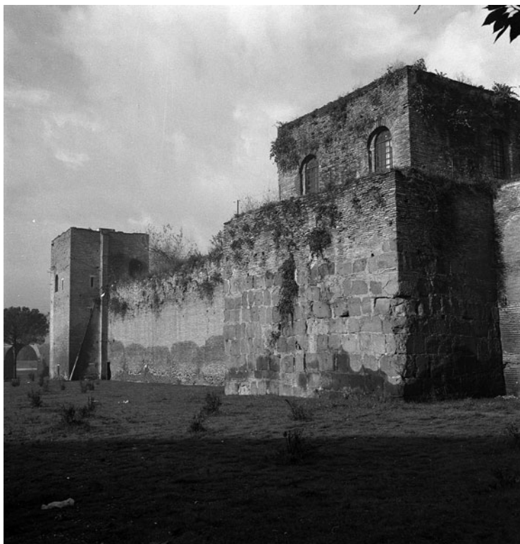
Fig. 10. Second tower east of the Porta Metronia in the Aurelian Wall showing the extensive use of reused blocks. (Photo by Ernest Nash. American Academy in Rome, Fototeca Unione Collection.)
