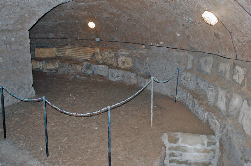
Fig. 4. Reused tuff blocks within the crypt of S. Laurentius in Lucina in the Campus Martius. (M. Andrews.)
