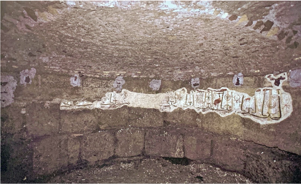
Fig. 3. Reused tuff blocks below the left apse of S. Angelus showing fragments of fresco. (After Meneghini and Santangeli Valenzani 2004, 81, fig. 60.)
