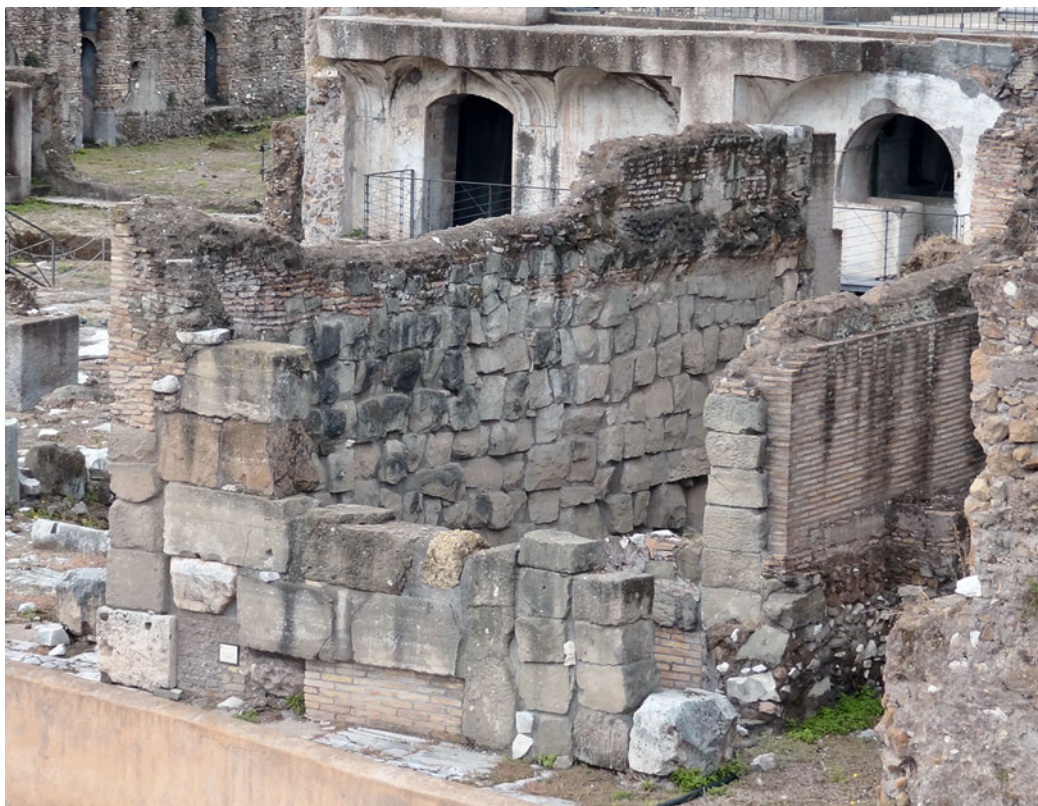
Fig. 15. A second domus solarata within the Forum of Nerva on the northern side of the early medieval street. The difference in the smoothed surface of the exterior (lower center) and the irregular appearance of the interior (upper center) is clear in this example. (M. Andrews.)
