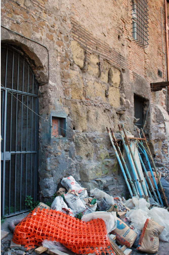
Fig. 7. Reused blocks on the northern façade of Ss. Quattro Coronati. (M. Andrews.)
