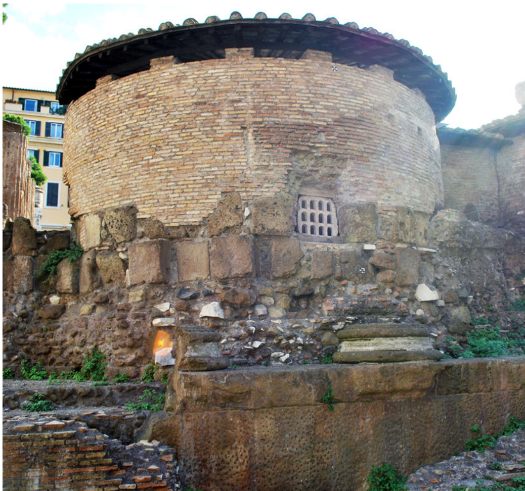
Fig. 16. Rear view of the apse of the small church of S. Nicolaus in Calcarario constructed on the podium of the Republican "Temple A" within the Area Sacra di Largo Argentina. Visible atop the podium are a lower zone of concrete and above it, a layer of reused tuff blocks with a small window of marble at the level of the crypt. (M. Andrews.)
