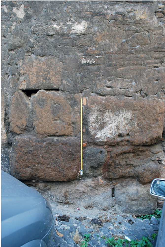
Fig. 6. Reused blocks in the lower level of the northern wall of S. Lucia (in Orphea), where they were used as infill. (M. Andrews.)
