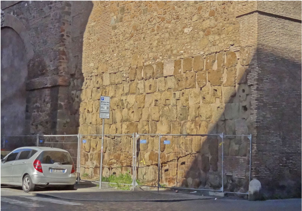
Fig. 11. Section of Leonine Wall west of the Porta Angelica with reused tuff blocks throughout much of the elevation. (M. Andrews.)
