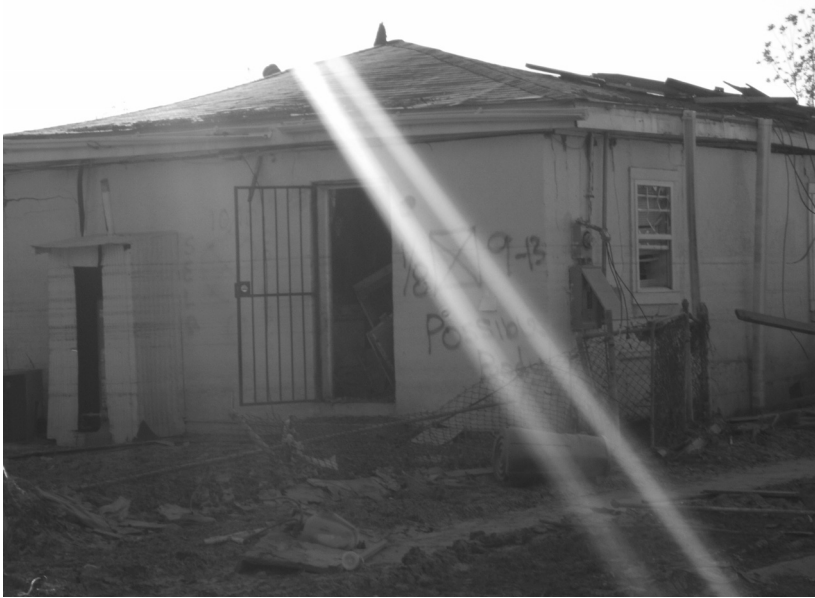
Figure 1 Katrina ruin in Lower Ninth Ward, New Orleans, October 2005. Photo by S. Dawdy.
