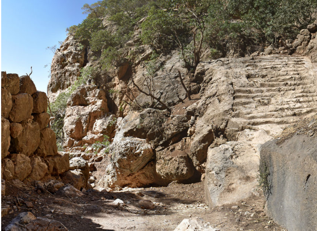
Figure 5. Wadi with northern terrace retaining wall (left) and main staircase (right), September 2022 (© Rabana-Merquly Archaeological Project).
