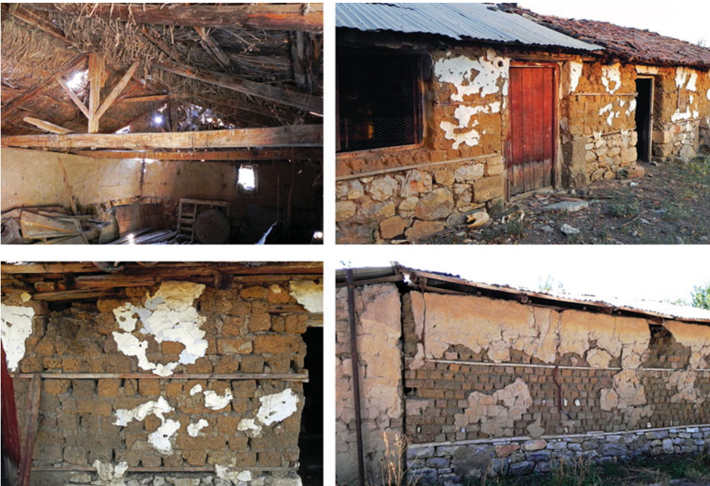
Figure 3. Abandoned storehouses constructed with stone foundation and a superstructure of mud brick at Neo Monastiri, Phthiotida, close to Koutroulou Magoula (photographs © Constantinos Papadopoulos).
