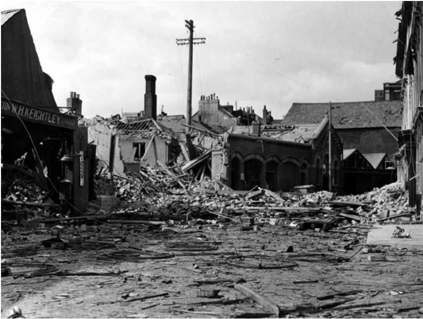
Figure 2. Bomb damage on Brunswick Street.
