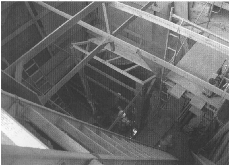
Figure 4. Looking down into the Middle Trench; the two archaeologists are excavating Trench D at the top of the Deep Sounding, protected from any debris falling from the face of the Middle Trench or from Trench M by the partially-closed sloping roof built of substantial timbers; looking south-east (photo: R. Rabett).
