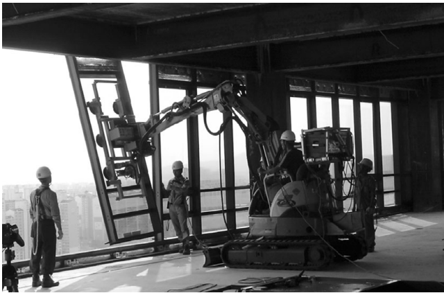
Fig. 1. ASCI (Automation System for Curtain-wall Installation).
