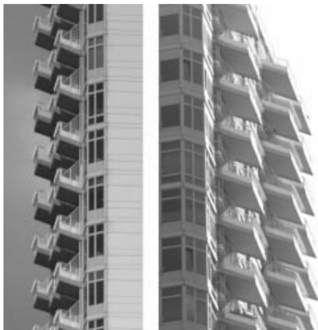
Figure 3 (Zaidi & Griffiths). (Left) A view of the apartment building “The Future,” located at 200 East 32nd Street in New York City. The balconies appear to tilt up, with tilt becoming more apparent the higher up the building one looks. (Right) The same building, but viewed from the opposite side. The balconies now appear to tilt downwards.
