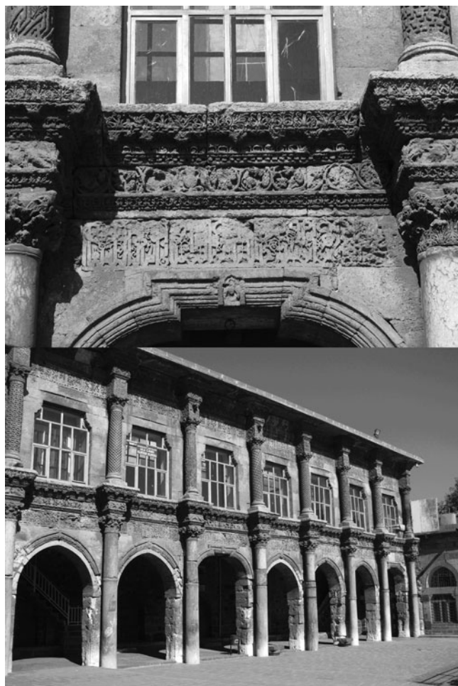
Figures 7 and 8. Late antique spolia reused in the western side of the medieval Great Mosque courtyard of Diyarbakir (Amida), Turkey
