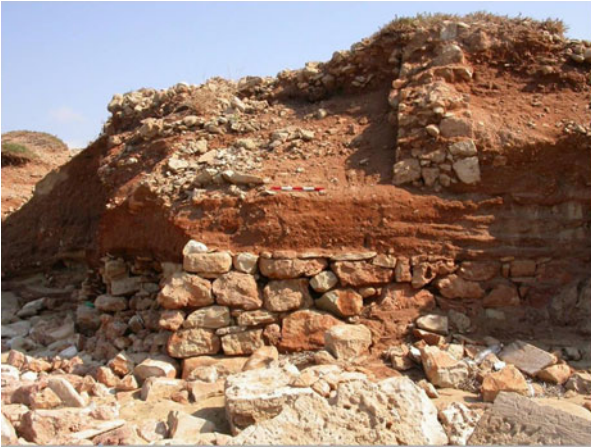
Figure 19. Coastal erosion at Tocra of the Greek city wall.
