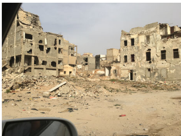
Figure 15. Houses on el-Shabi Street, behind the Suq el-Hout (Fish Market).
