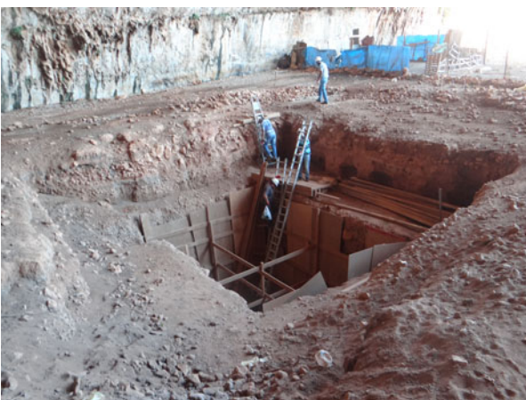
Figure 7. Timber shores.
