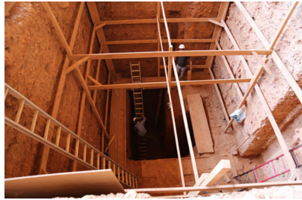
Figure 8. Removal of the timber shores.
