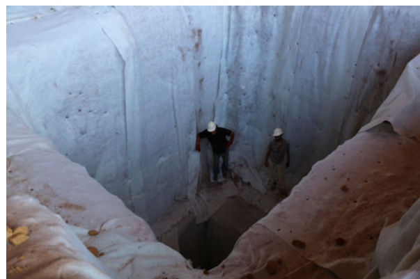
Figure 9. Lining the sides of the excavation with the geotextile.
