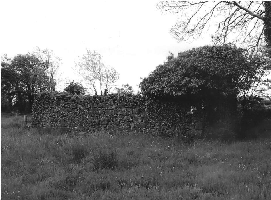
Figure 2. Burke/Fannon house in Kiltreevan, County Roscommon, built with stone walls, thatch roof, two-to-four rooms, two windows in front, six living therein, as listed in the 1901 Irish census. Photograph courtesy of Ted McGraw.
