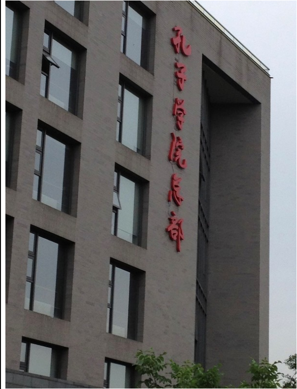
Hanban headquarters. Photo by J. Hubbert
